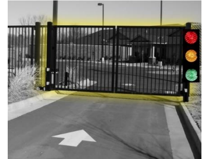
Figure 4-VIII: Illustration of a gated entry with traffic lights securing a confined area.
