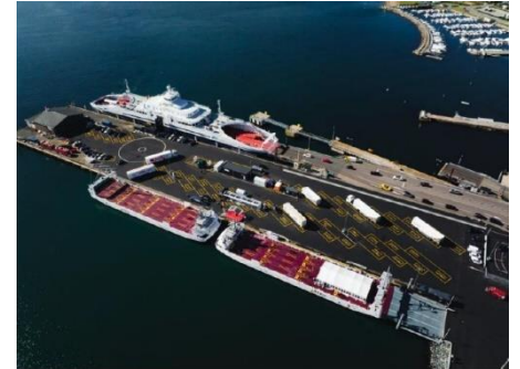
Figure 4-IV: ASKO sea drone port at the Port of Moss.
