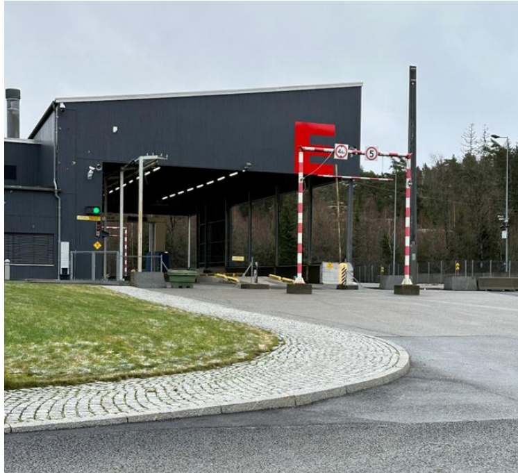
Figure 3: Vehicle scanner at Svinesund Customs station.
